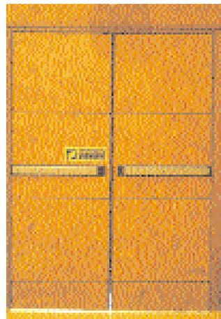
**Hall walls must be detailed for safety and without protrusions. A panelled treatment helps to integrate the door and wall surfaces. This example of an escape door has neat push pads instead of the usual panic bar.**
