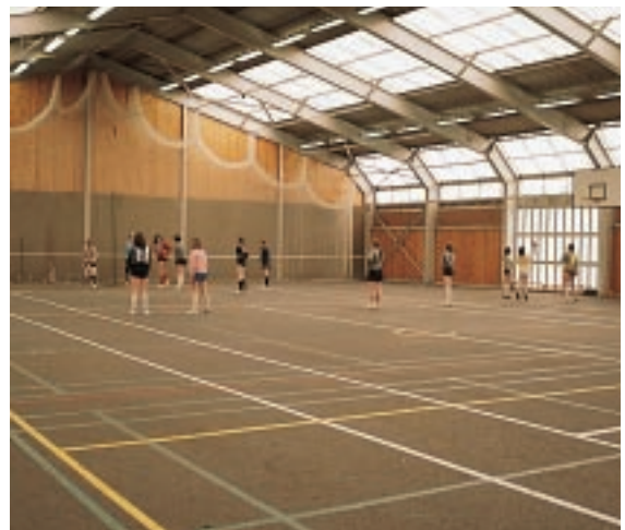
A first generation sports hall with lighting and structure that would be difficult to upgrade to meet current standards.
